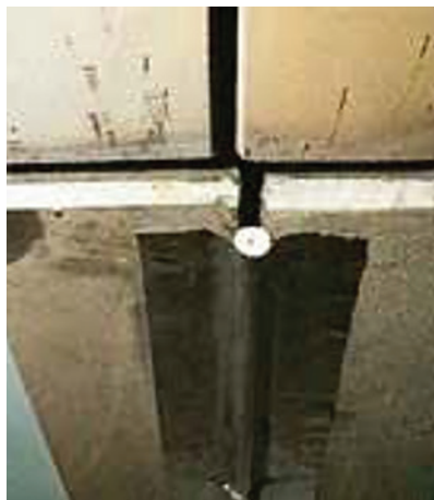
Cylindrical ceramic OK Backing Pipe 12 in use in bridge construction. Process: MAG
