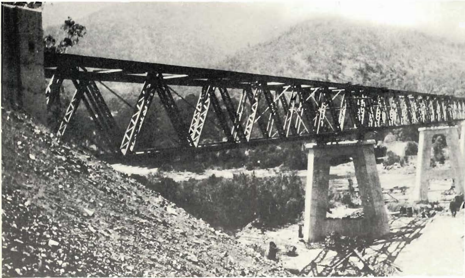
The 750 ft. long Mackillop Bridge over the Snowy River in 1932 had world's second longest welded spans. Floods washed it away soon after it was opened.
