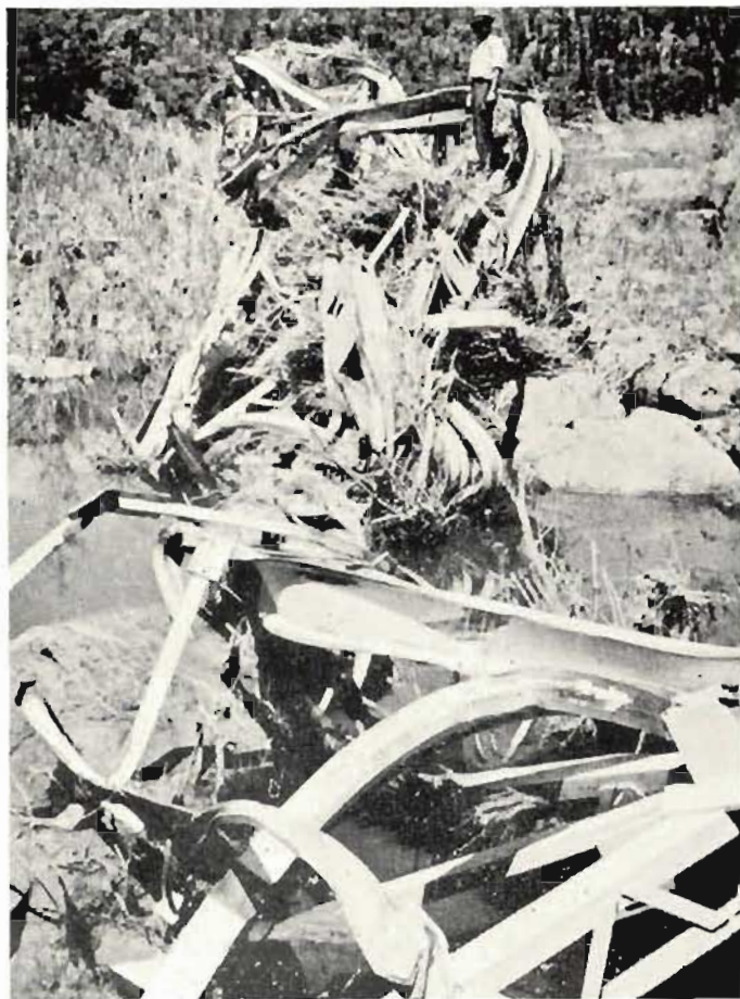
Mackillop Bridge wreckage (left) showed that all welded joints had stayed intact.
