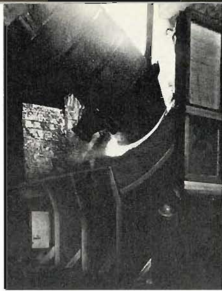
BOS furnace is tilted and charged with scrap. Transfer ladle is then emptied into it.
