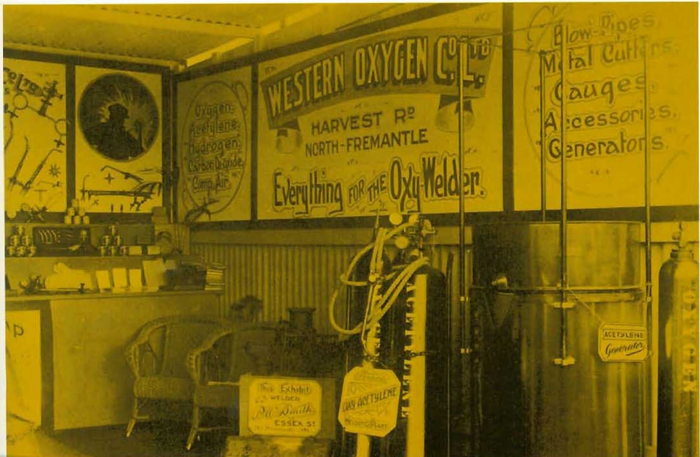
Low-pressure acetylene generator at right of the picture below was part of a Westox exhibit at a Perth show in the early 1920s.
