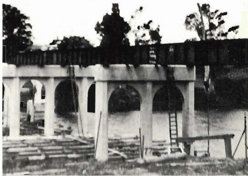
Welded plate girders were used for Tambo River Bridge (below) in Gippsland about 1930.
