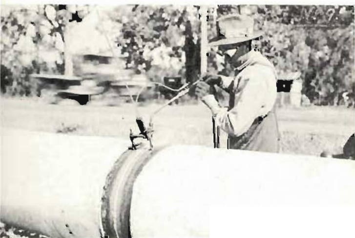
Linde oxy-acetylene pipe welder was the most efficient of all welding systems in the repair of Perth-Kalgoorlie pipeline in 1930s.
