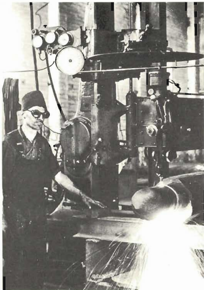
Crab for 100-ton crane was welded at Ruwolt's without jigs or positioners.
