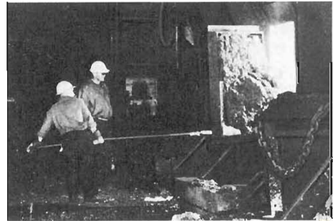
After 20 minutes, "blow" is turned down and steel sample taken for speedy analysis.
