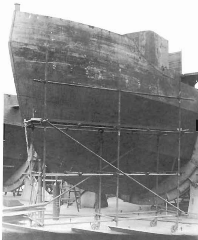
Wartime construction of small ships in turning cradles enabled difficult overhead welding to be reduced.
