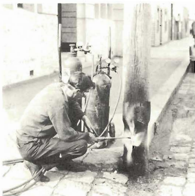
Charring of power and telegraph pole bases with oxy-acetylene torch helped prolong life of the poles.
