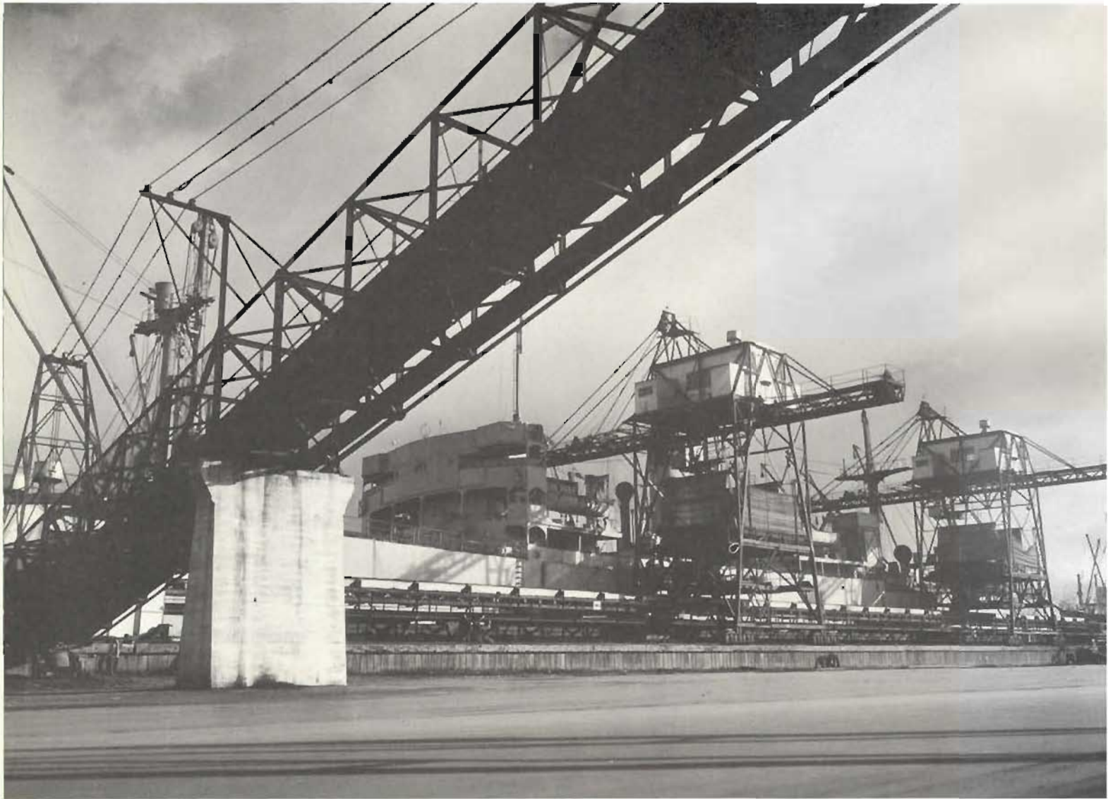
Welded 100-ton grab bucket unloaders were designed and built by Malcolm Moore for gas companies in Melbourne and Sydney in early 1930s.
