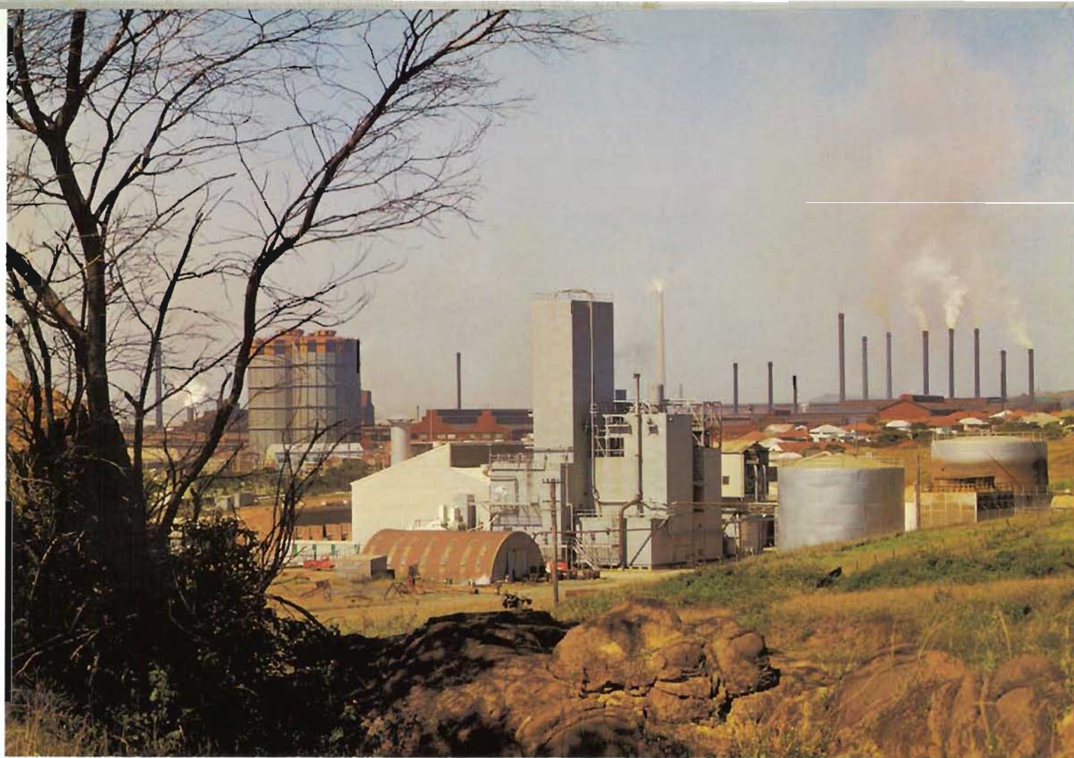
C I G 's tonnage oxygen plant at Port Kembla. Steelmills are fed from it by pipeline.
