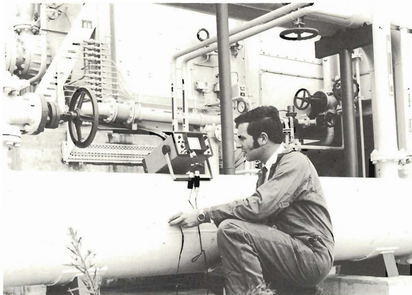
Ultrasonic weld testing of a process pipeline at a Sydney chemical plant.
